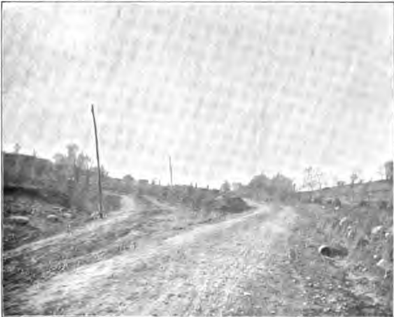
Independence road, Warren Co., one-half mile west of Hackettstown, after improvement. Showing changed line to avoid steep grade.
